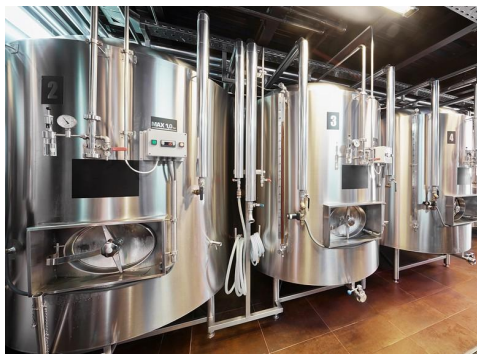
Figure B3. Fermentation tanks.
